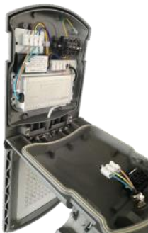
Re-fit light unit
